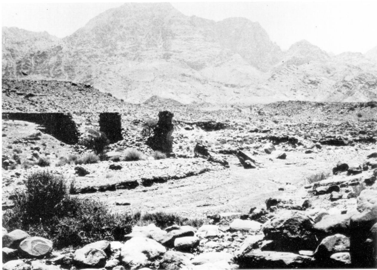
Pillars of aqueduct bridging Wadi Jeko at Fenan, Jordan
