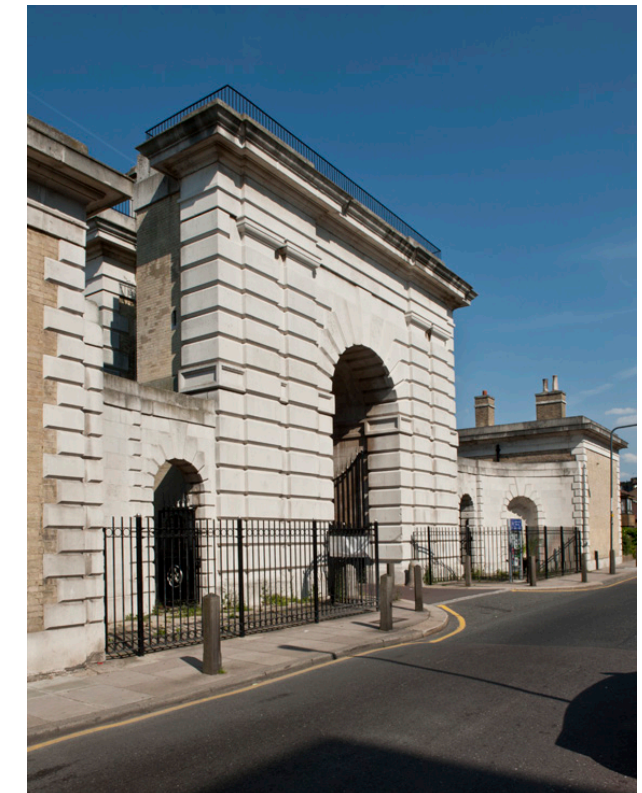
386. Cambridge Barracks entrance arch and lodges, Frances Street, 1847–8, from the west in 2010
