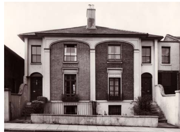
392. Nos 118–120 (Albion Cottages) of 1843. Photographed 1953
