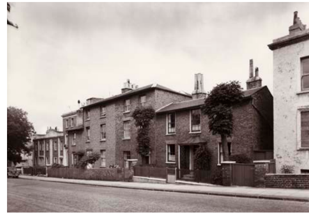
390. Nos 143–159 from the south-west in 1962 (right to left): No. 159 (Anchor Cottage), 1826; Nos 155–157, 1835–9; No. 153, c.1830; Nos 143–151, 1843
