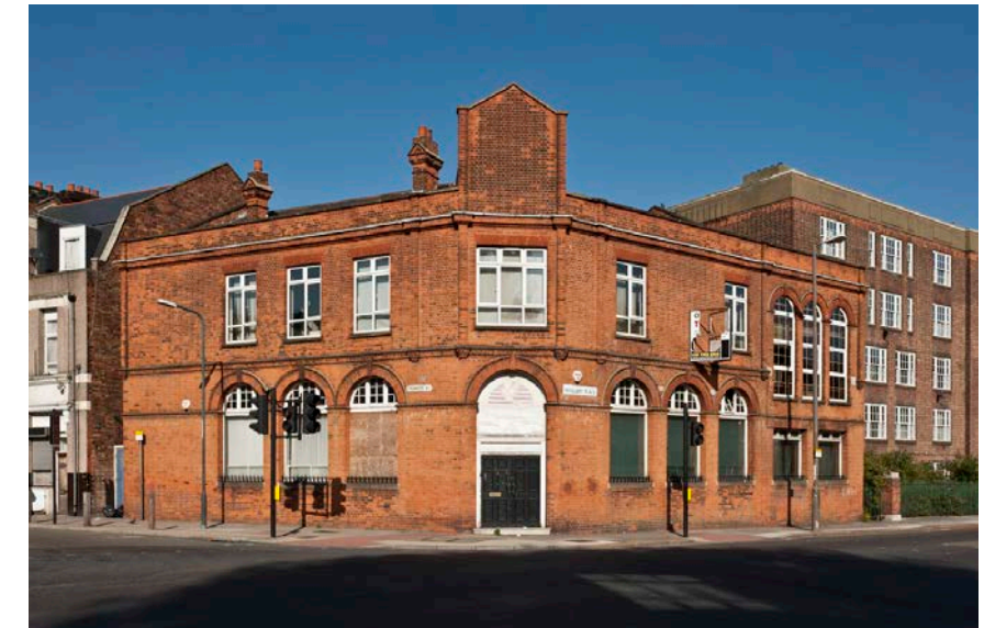
402. 1 Artillery Place, 1903–4, shop and workrooms for Joseph Daniels and Co., military tailors and outfitters. Also showing (right) part of Cambridge House, 1937, married soldiers' quarters. From the south-west in 2010
