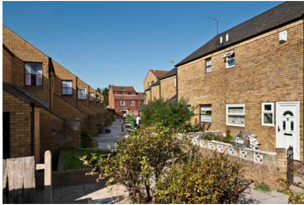
407. Whitby Road, Red and Cambridge Barracks Estate, 1979–83. For Greenwich Council. From the south-east in 2009
