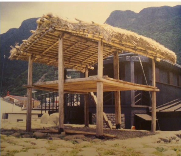
Figure 24 New Ta'u demonstration house with traditional tagaka –cool house feature, 1997
