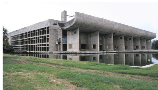
Figure 17 Le Corbusier’s Palace of National Assembly-Chandigarh, India is perhaps his best known building built within his master plan
