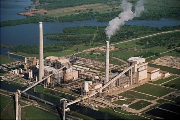
Figure 2 Aerial view of Power Plant- San Antonio, TX, USA, 2009
