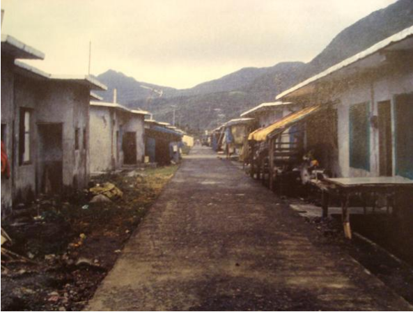
Figure 22 Government-built concrete barracks on Pongso-No-Tau Island, Taiwan
