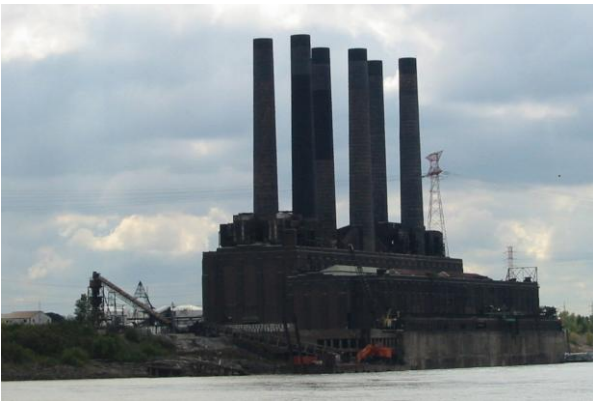
Figure 3 Abandoned riverside power plant- St. Louis, MO, USA, 2005
