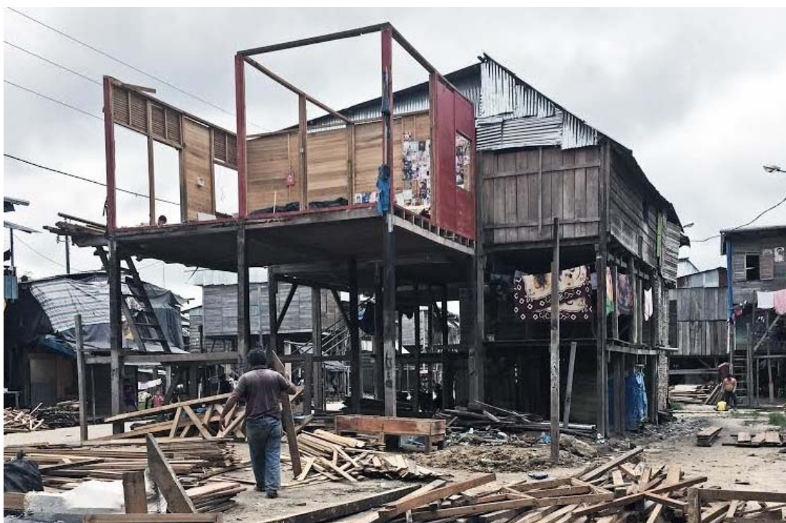
Figure. Demolition of the house in Bajo Belen. Courtesy CASA team.
