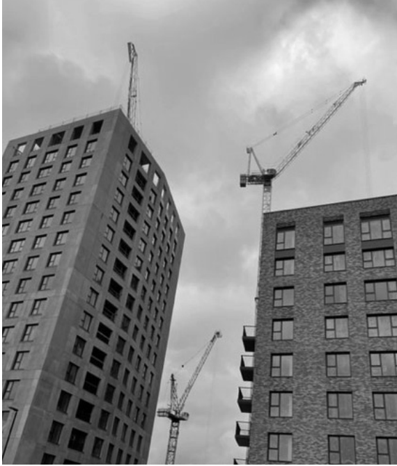
Image 6: New developments being built in Coventry Cross. Abdul 2021
