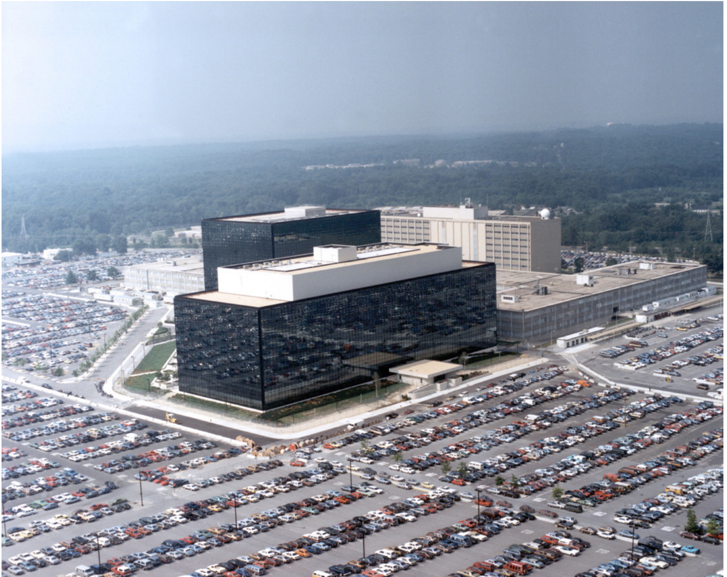
Headquarters of the NSA at Fort Meade, Maryland.
