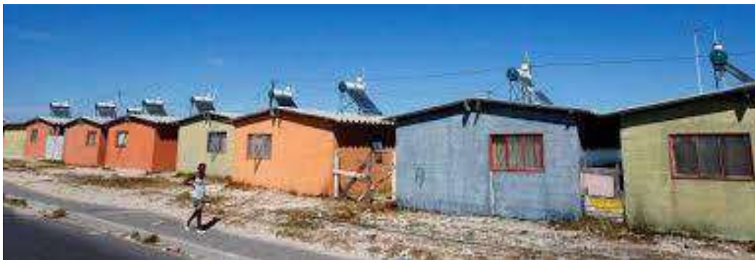
Figure 4: Roof top solar water heater in Joe Slovo
