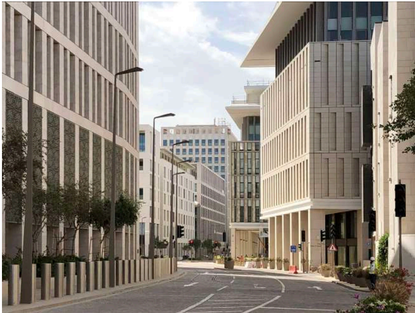
Figure 5. Msheireb, Doha, Qatar
