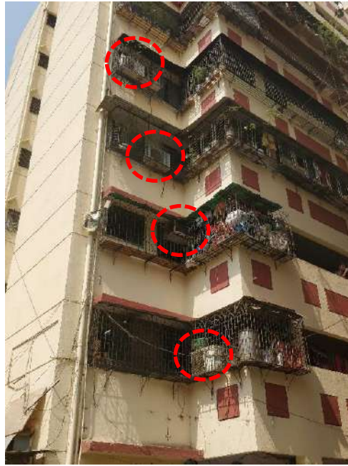
Figure 2: Installed air conditioner in SRH
