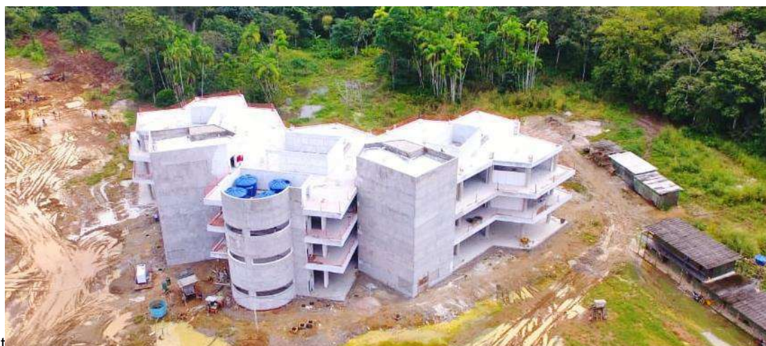
Figure 6: The pedagogical block under construction in the Atlantic Forest (jun/16)
