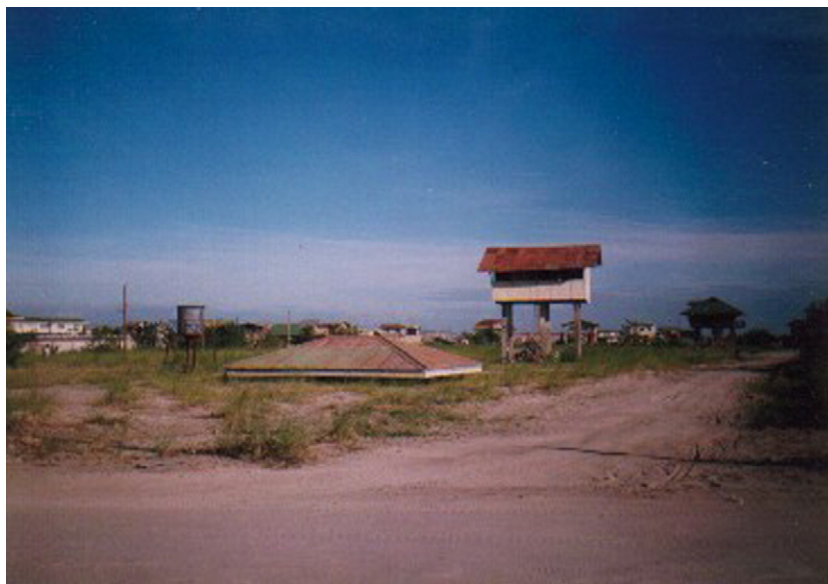
Fig. 4. Houses raised on concrete posts in Cabambangan, Bacolor, in December 1997 (photograph by J.-C. Gaillard).
