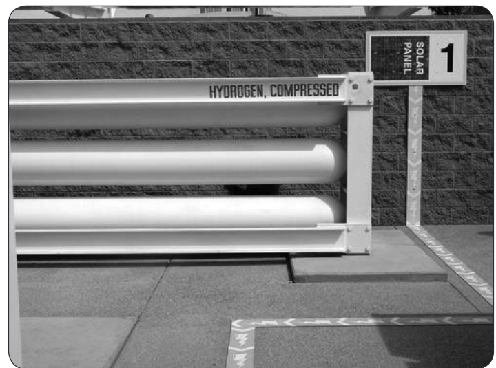
Image courtesy of DOE/NREL, photo credit Keith Wipke Hydrogen can be stored in high-pressure tanks.
